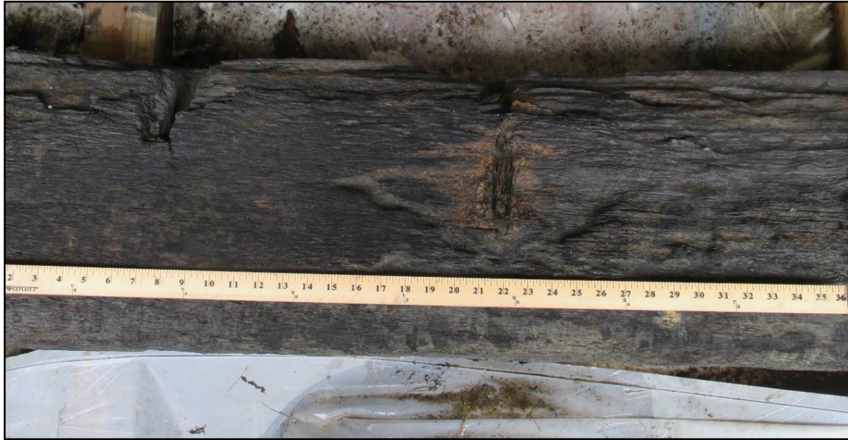
Figure 78. Exposed drift pin at the edge of the keel.
